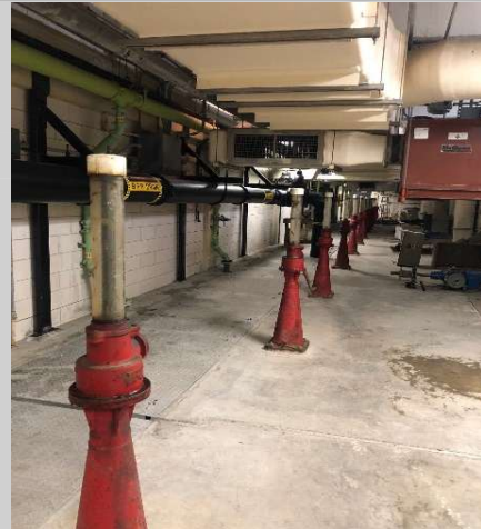
Primary Clarifier Influent Building
