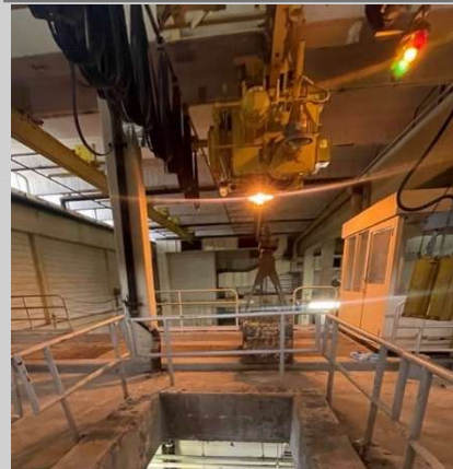
Grit Crane Loadout
