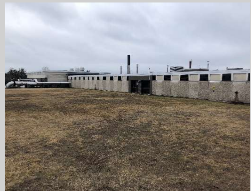
Secondary Clarifier Influent Bldg & Odor C
