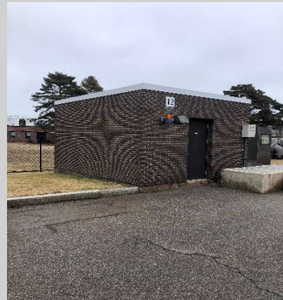
Salem Neck Pump Station
