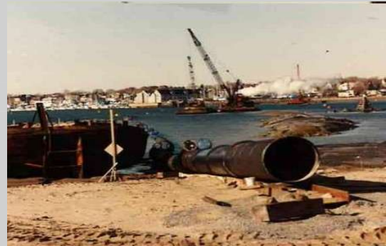
42-inch Beverly Force Main Being Installed in 1984.
