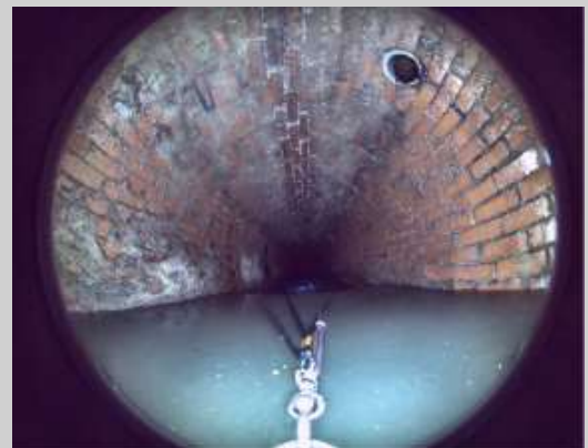
46 x 48 Brick Horseshoe Sewer in Walnut Street
