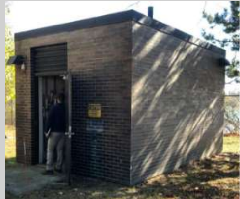
Beverly Metering Station
